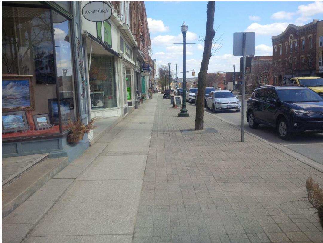
Photo 1 – Existing sidewalk configuration with 1.5m concrete sidewalk, banding, and paving stone blvd
