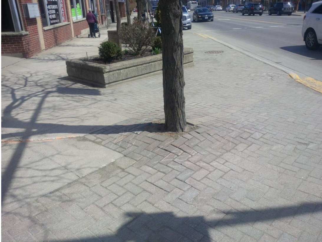
Photo 3 – Paving Stone heaving around tree
