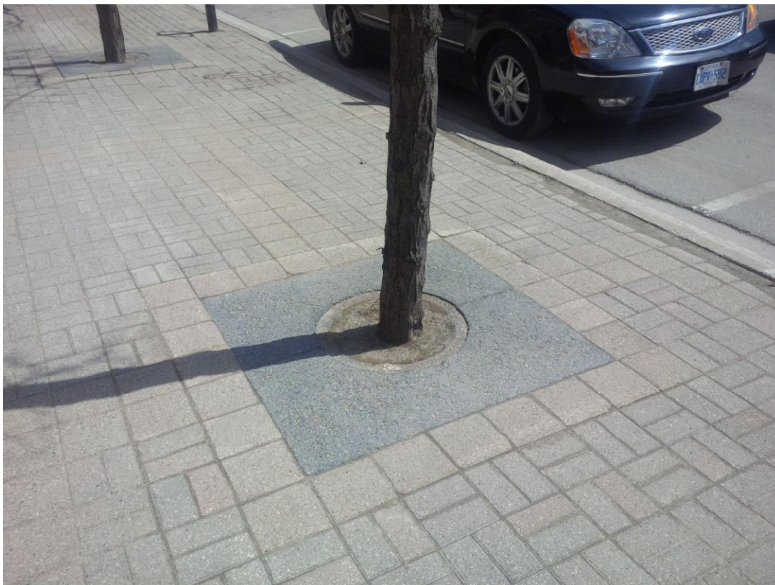
Photo 4 - Tree with original tree grate and no heaving
