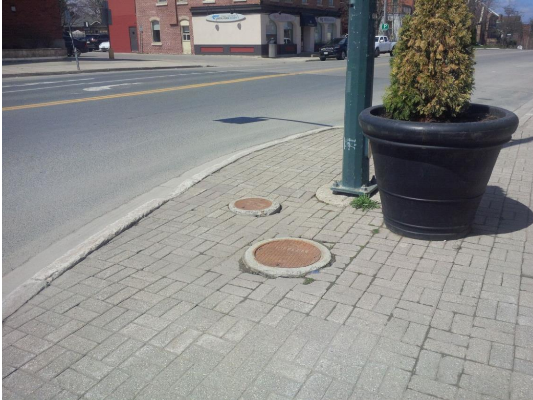
Photo 5 – Settlement around junction boxes
