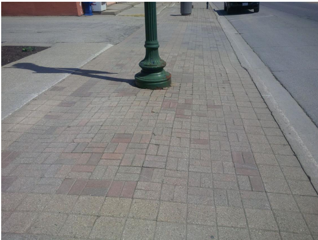
Photo 6 – Uneven and broken paving stones
